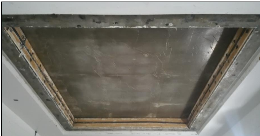
Receive Room View of Test Specimen Installation
